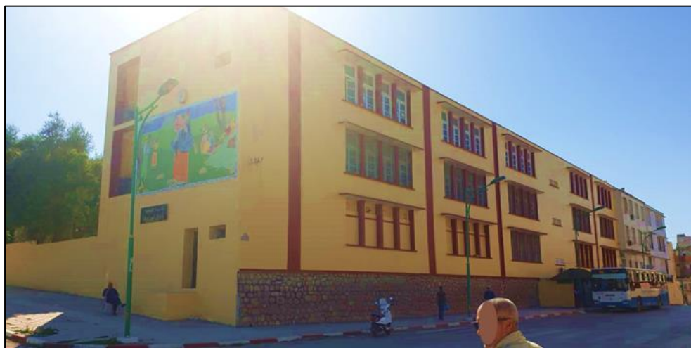
Figure N° 05: 'Tarek Ibn Ziad' urban school after rehabilitation. (Source: Lamari & Lazri, 2021)
