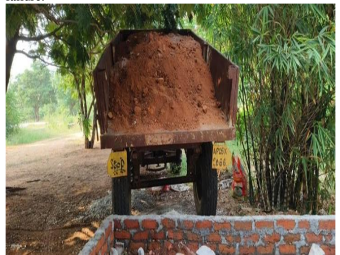
Figure 3: Refilling and Compaction of soil
